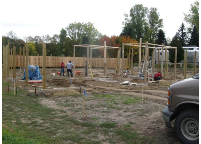
The Bonsai and Penjing Garden takes shape. Construction continues with the framing of the structure within the garden. 10-2-12
